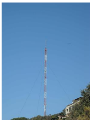
Antenna radio RAI Camaldoli - Napoli
